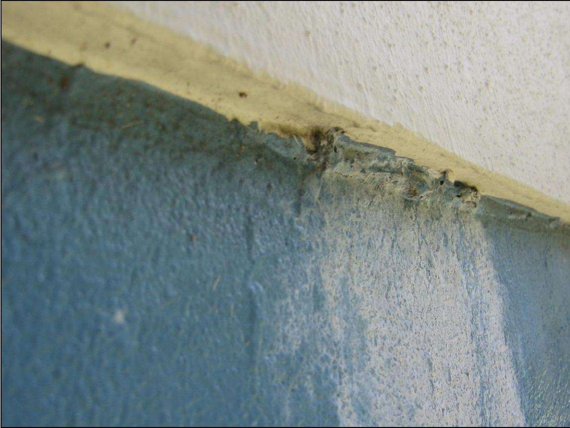
Photograph 2: Efflorescence at Accessory Joint
