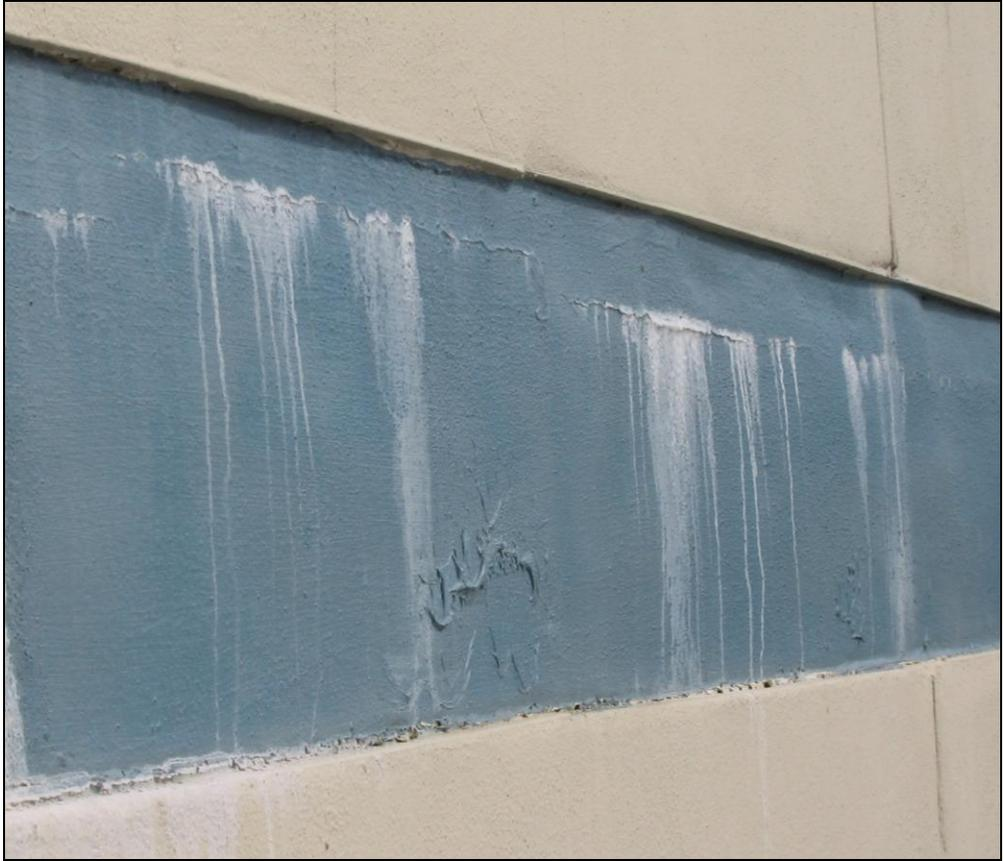
Photograph 1: Efflorescence Due to Water Seeping Through Stucco
